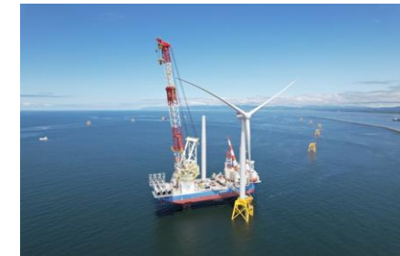
<Turbine Generator Installation>
